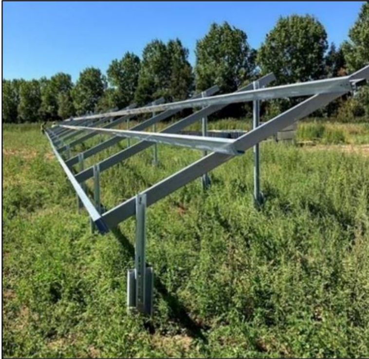
Plate 3.12: Example construction piling for the installation of the Solar PV mounting structures
