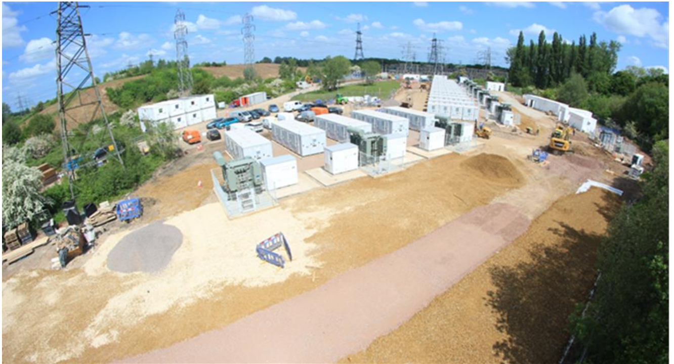
Plate 3.10: Example of the Construction of BESS Compound
