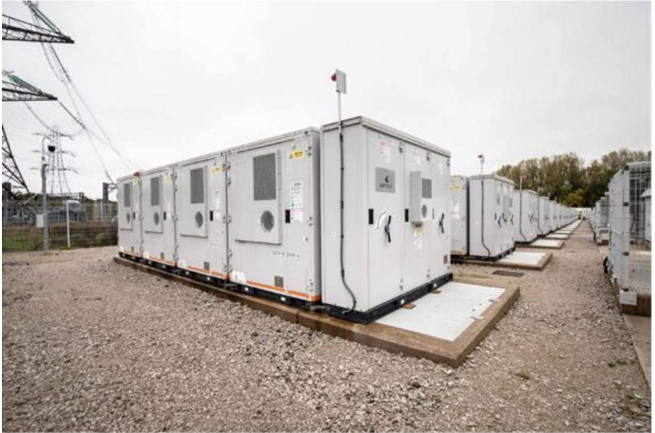
Plate 3.9: Example of an Operational BESS Compound
